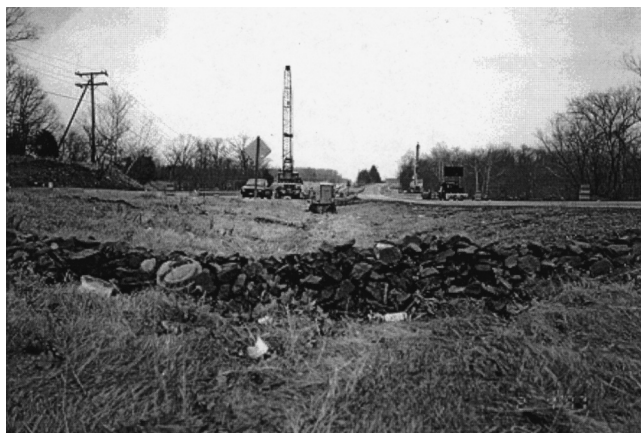
FIG. 2. Goose Creek Swale and Check Dam System
