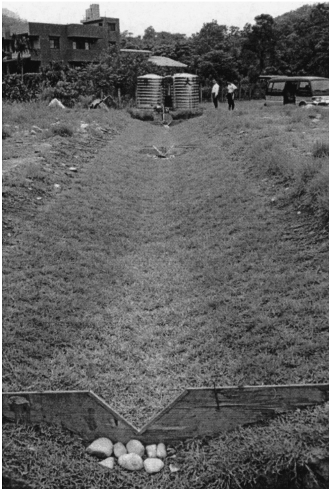
FIG. 1. 30 m Test Swale with 1 Check Dam at Taiwan Site
