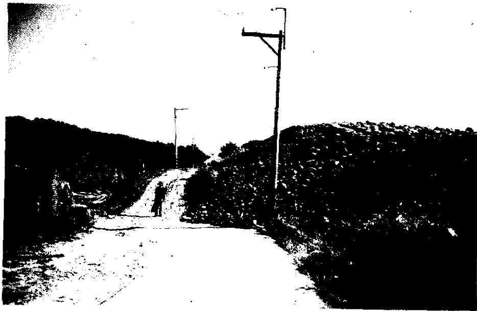
Figure 3. At this location on the north embankment along the Choshui River, the road obviously shows a horizontal offset of 1.9 m caused by left-lateral thrust faulting.
