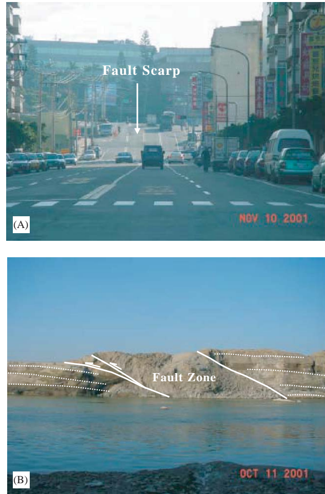
Fig. 9. (A) Photograph of the fault scarp of the Hsinchu Fault in Hsinchu City. The foundation excavation of the far building in hanging wall showed upright and brecciated bedrock, which is the only field evidence of the Hsinchu Fault. (B) Photograph of an outcrop of the Hsincheng Fault along the Touchien River. White dash-lines represent the bedding. A low angle thrust with vergence to the west reaches the ground surface with a fault zone of 4–5 m in width that is bound by two slip planes. The hanging wall is composed of Pliocene coastal deposits, sandstones and shales, while the footwall is the younger (Pleistocene) sandstone dominant unit that is believed to be the distal part of an ancient fan-delta created in the mountain front.
