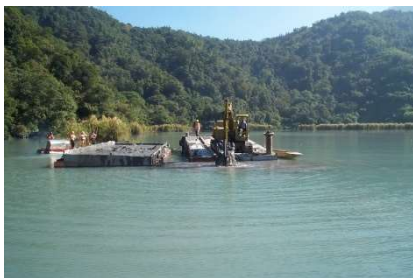
Figure 2.5 Dredging by excavator in 2006
