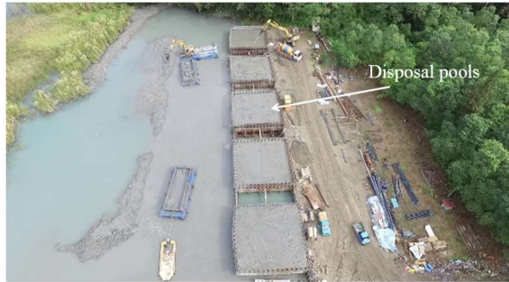
Figure 2.8 Sediment disposal site in 2017
