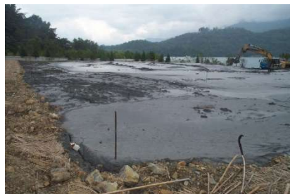
Figure 2.7 Sediment was placed at Sun Moon Lake nearby for engineered fill in 2006
