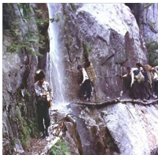
Photo 1.1 A look at materials and equipment being carried during the reconnaissance of the Kurobe River.
