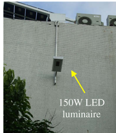
Fig. 20. 150 W LED in solar roadway lighting system.
