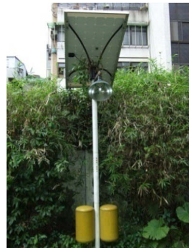
Fig. 15. 18 W solar-powered LED lighting system.
