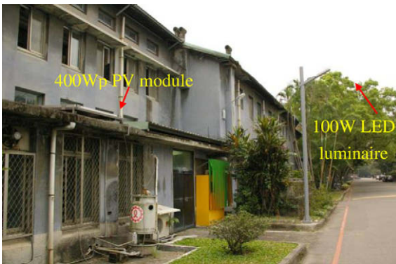
Fig. 18. 100 W solar-powered LED roadway lighting system.
