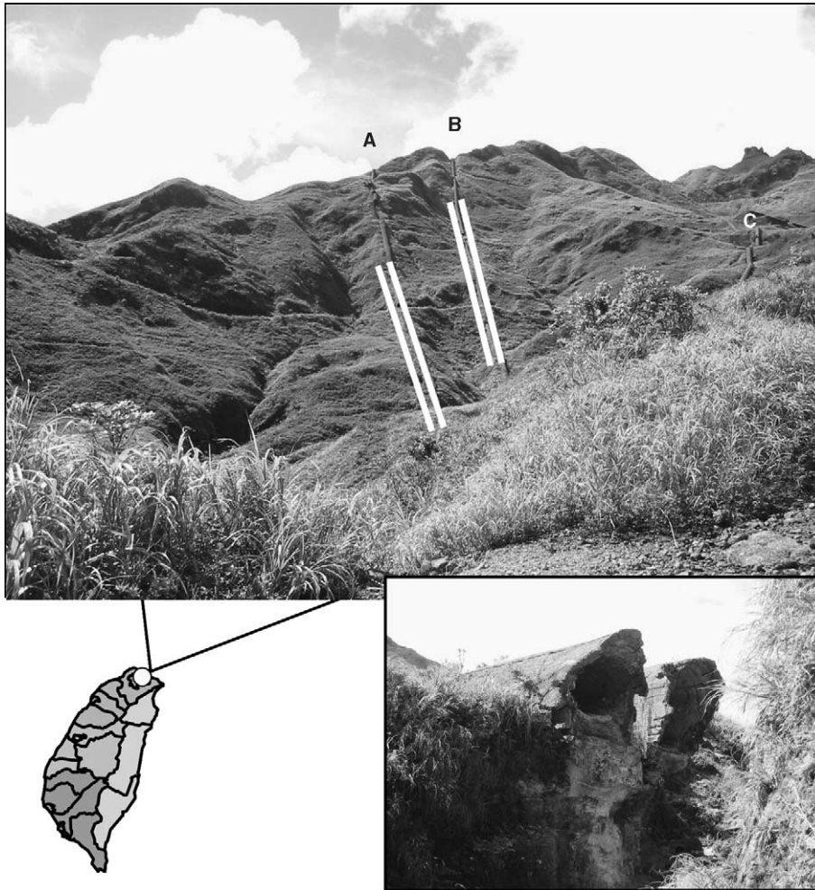
Fig. 1. Site view of tunnels for discharging exhausted flue gas from a copper smelter plant. Samples were taken from the bold-faced sections.
