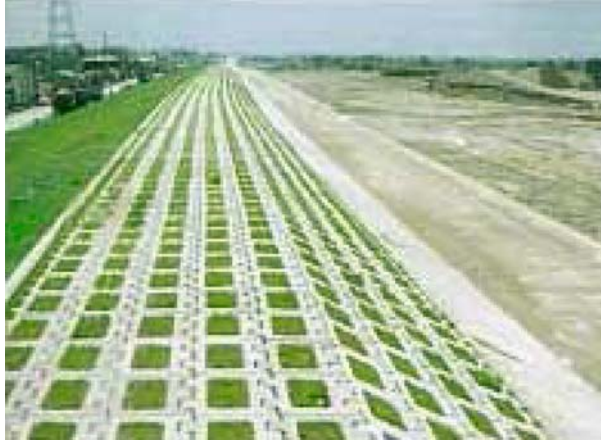
Figure 5. Dike construction employing ecology methods.
