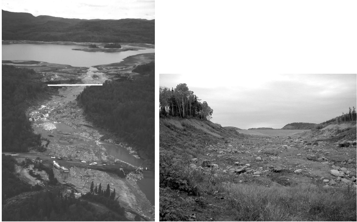
Figure 16. Vicinity of the failed dyke which triggered the geomorphic flood of July 1996. Left: helicopter view of the situation immediately after the flood (photo courtesy of Dr. G.R. Brooks, GSC). Right: ground view of the situation in September 2000 (photo by H. Capart). The position of the original saddle dyke is shown in white on the left photo.
