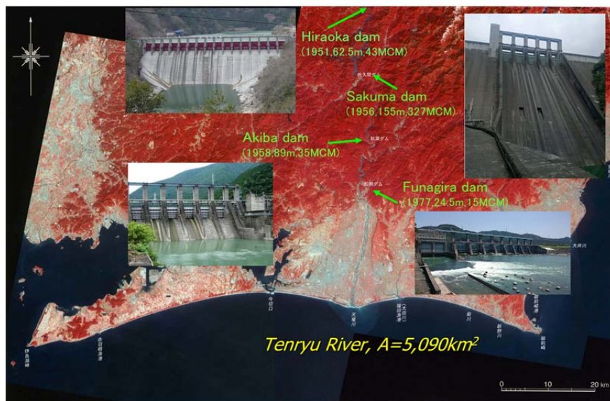
Figure 3 Downstream area of the Tenryu River and cascade hydropower dams
