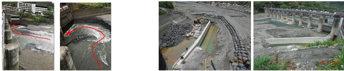
Abb. 11: The previous hydraulic behavior Abb. 12: Build the diversion wall of the sluiceway
