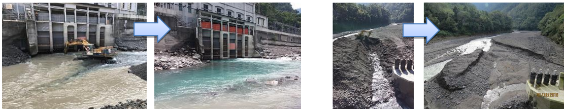
Abb. 14: Dredge by mechanical excavation. Abb. 15: Longitudinal or Lateral Erosion Enhancement.
