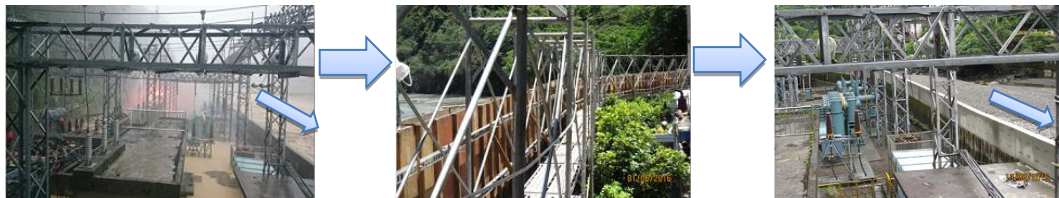
Abb. 10: Heighten the flood wall to prevent flood.
