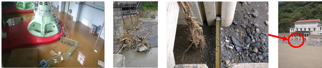
Abb. 7: Impacts of sediment disasters on hydropower facilities.
