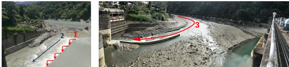
Abb. 13: (1) (2) Hydraulic head makes the ditch in river channel when opening the sluiceway gate. (3) Water flow can be directed straight to flush the sediment in front of the water intake.
