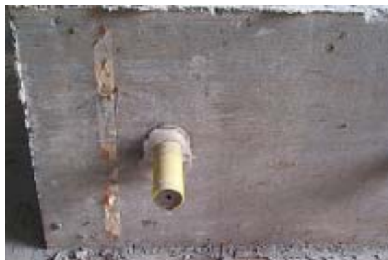
Figure 8 Appearance of SCC-00 (SCC, no vibration)
