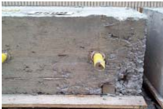
Figure 7 Appearance of HPC-00 (HPC, no vibration)
