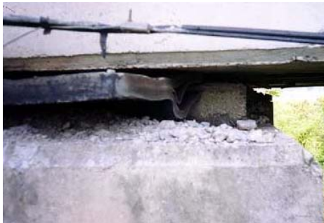
Figure 3. Bearing damage on Yeng-Feng bridge in Chi-Chi earthquake (sliding out of the pad seat)
