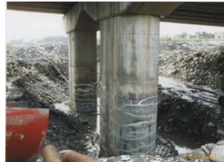
Figure 3. Bearing damage on Yeng-Feng bridge in Chi-Chi earthquake (sliding out of the pad seat)
