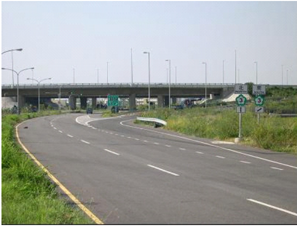
Figure 1. The Wu-Zi highway bridge.
