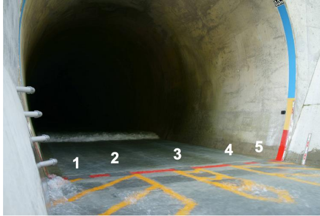
Figure 2 Koshiibu SBT outlet with five IPs for bedload monitoring
