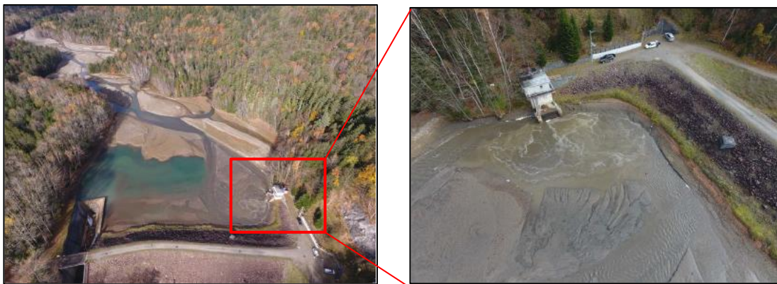
Figure 2.The intake of Horoka hydropower plant when water level was 2.6m (2018.10)
