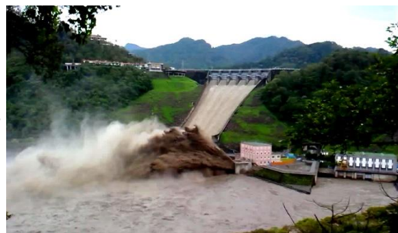
Figure 9. Photo showing muddy water sluiced out from the sluice tunnel as the density current reached the dam.
